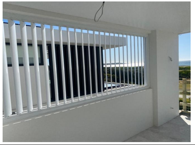
Vertical operable 150mm louvres in a 50 x 50 frame
