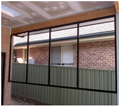
Welded 50x50 Frames
