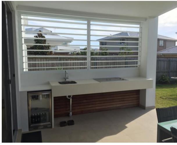
Horizontal Operable 150mm louvres in a 50 x 50 frame
