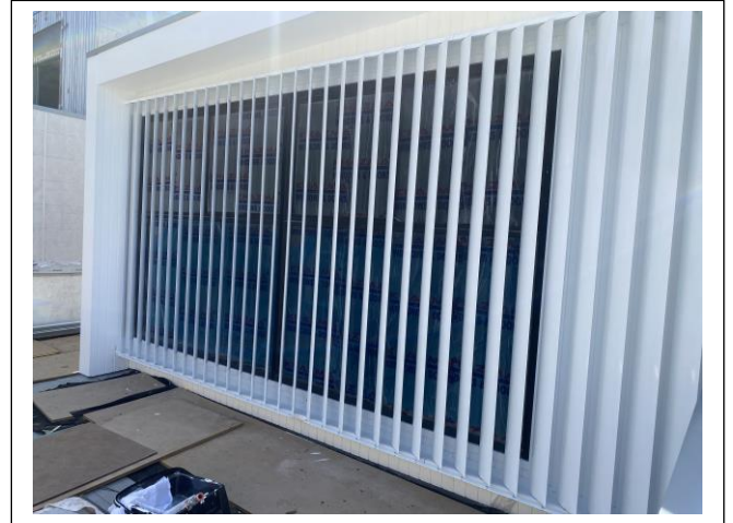
Vertical operable 150mm louvres NO welded frame
